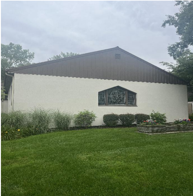
Front of Church – Facing East
