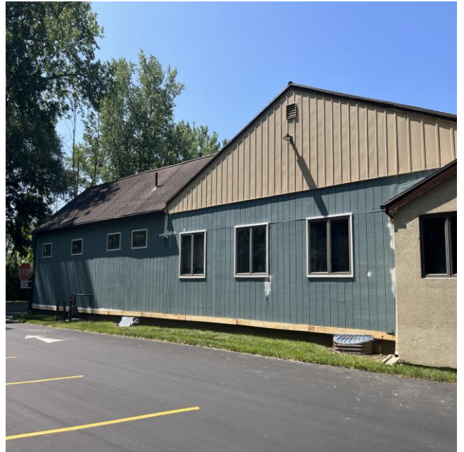
Beginning to Paint the North Side of Church
