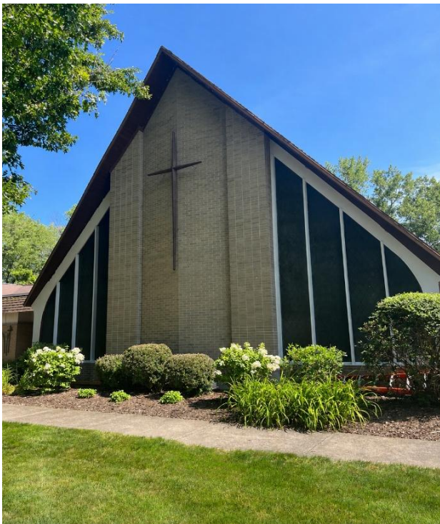
Front of Church – Facing West
